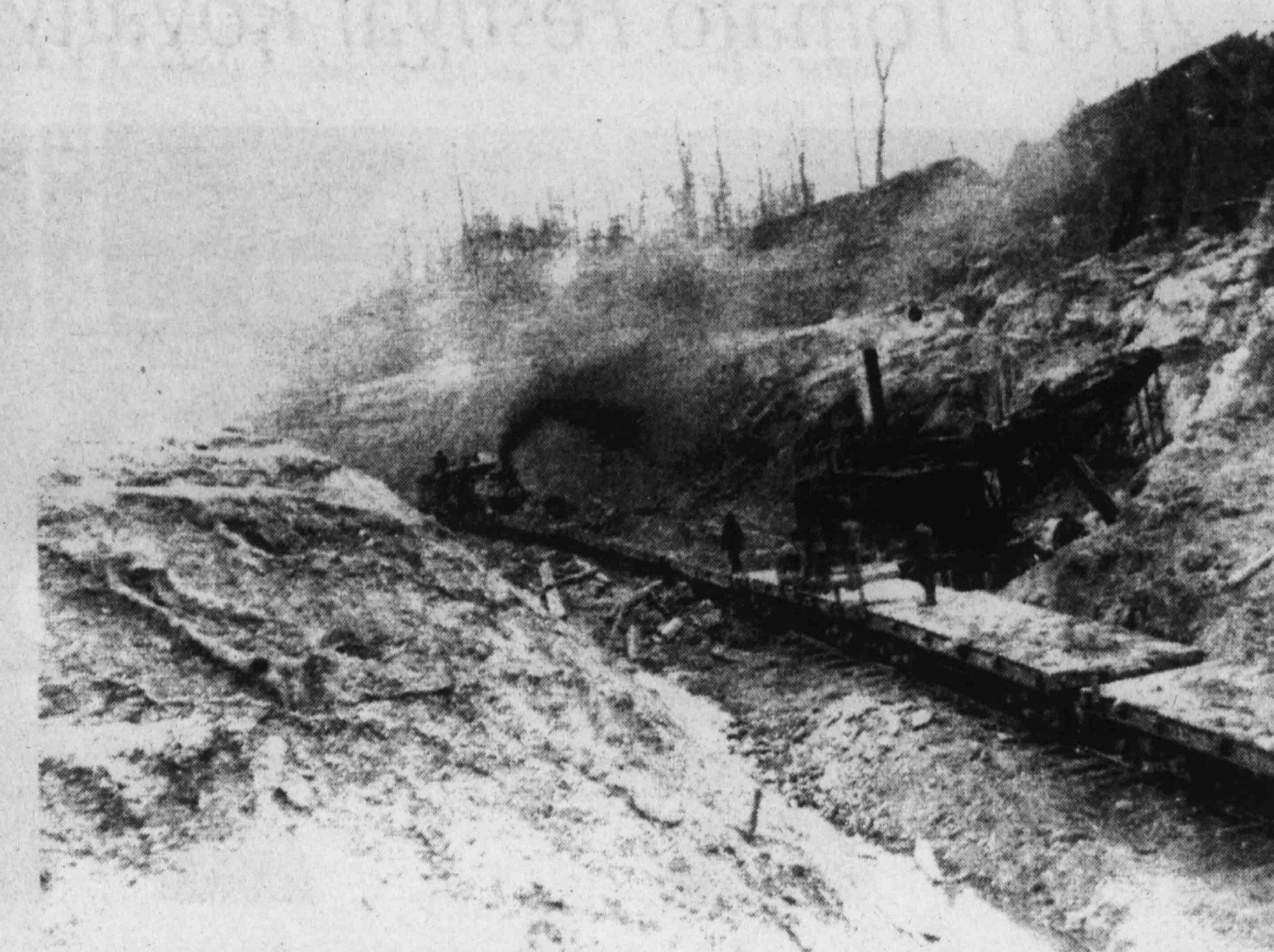
RAILROAD CONSTRUCTION on the rails at Curve.
